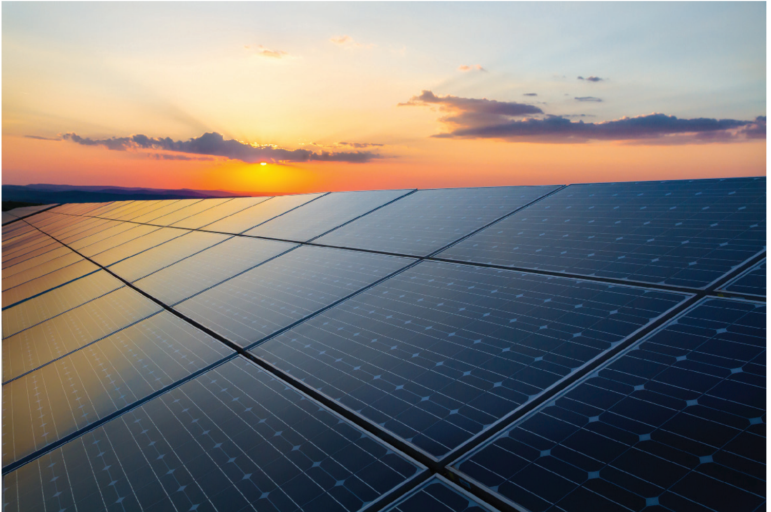
Community solar, a new offering for Illinois, will begin construction across the state this year.
