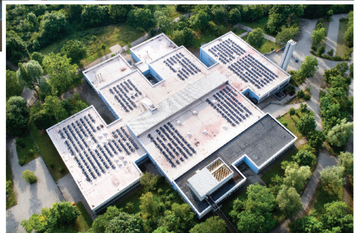
Applying solar to vacant roof space is a great way to increase property value and decrease operating expenses.
