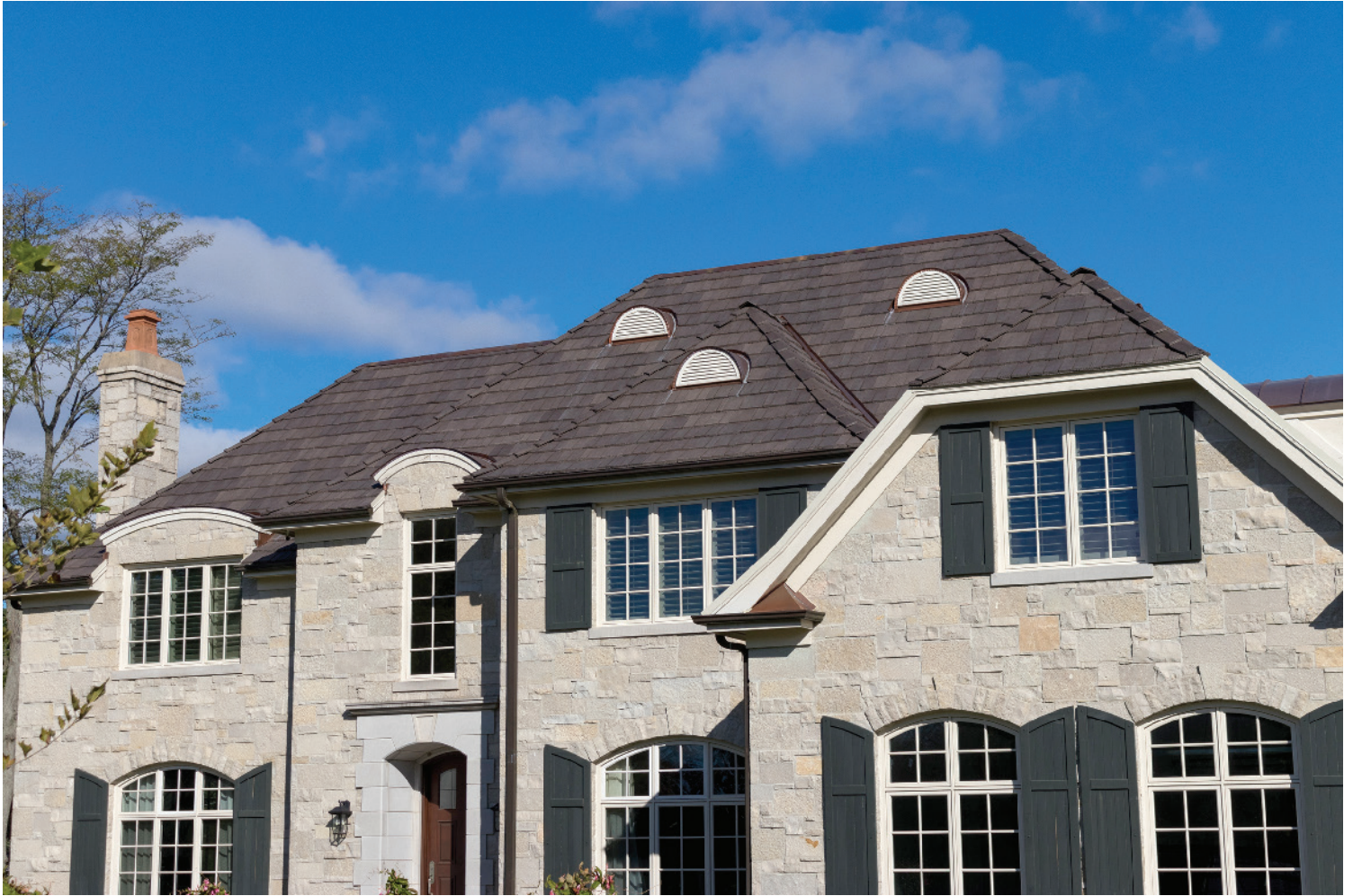
The Mayberry's home showcases a new DaVinci Roofscape installed by Shake Guys.
