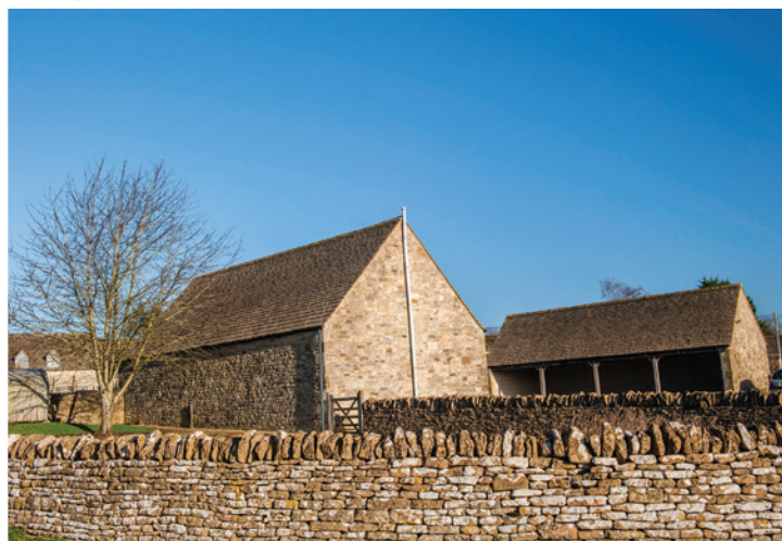
Farm buildings in Great Barrington.
