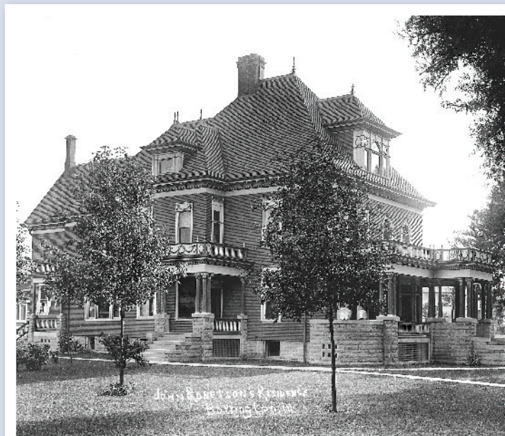
The John Robertson, Jr. home was renovated in 2013-15 and is now known as Barrington's White House.
