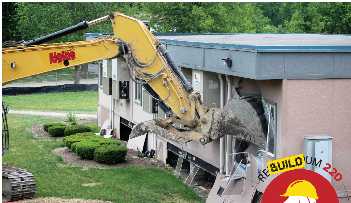
Construction crews tear down the mobile classrooms at Station Middle School on June 7, 2021.
